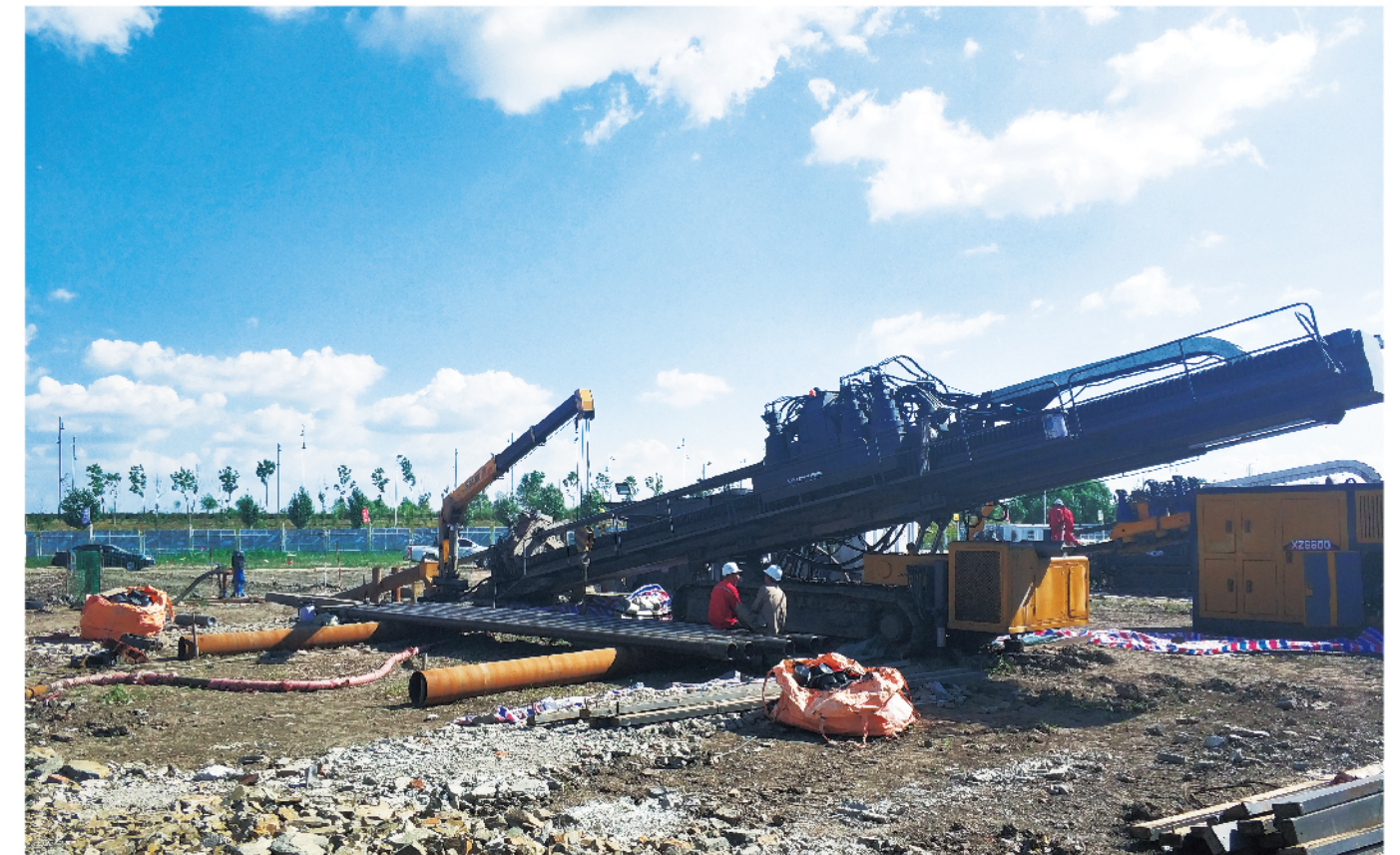
XZ6600 working for the 3 km water supply pipe project with a diameter of 813 mm across the Songhua River
