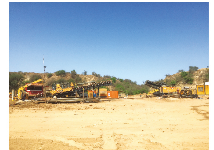
XZ6600 working for crossing the mountains in India
