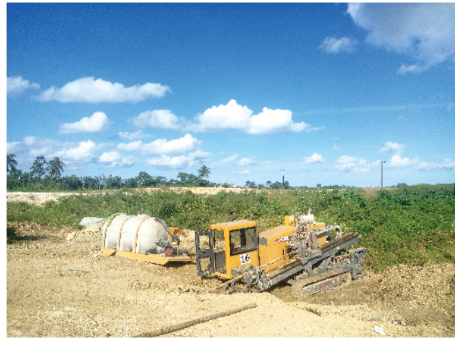
XZ320D working for power pipeline construction in Cuba
